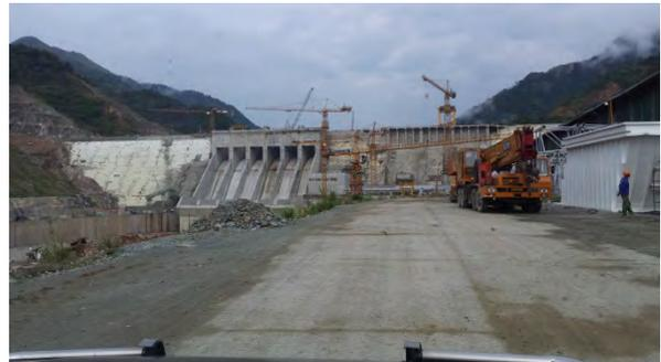
Damwatch instrumentation expert Alan Sutherland has recently been on site to inspect progress of the instrumentation system at Lai Châu Dam in Vietnam during reservoir impounding. Alan is the instrumentation specialist on the design team for the 137m high Roller Compacted Concrete hydro power dam, which will generate 1200MW. For more information contact Tony Harker at [tony.harker@damwatch.co.nz](mailto:tony.harker@damwatch.co.nz).
